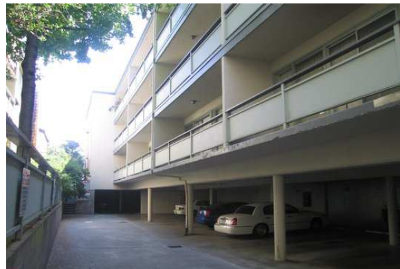
Figure 2. showing use of Soft storey in buildings
