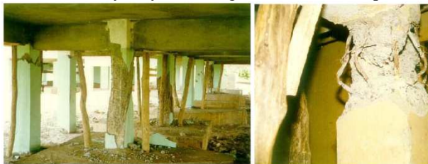
Figure 4. Damages in columns during earthquake
