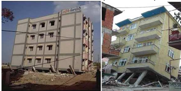
Figure 3. failure due to large lateral displacement in soft storey
